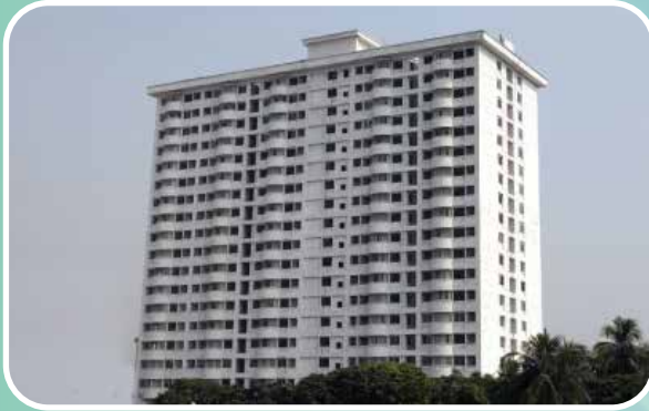
Project Name: Residential Tower Building of Police on Turnkey Basis
