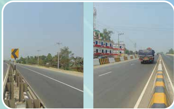
Project Name: Construction of SASEC 4-LANE ROAD PROJECT, CONTRACT NO-3, DULLAMARI ROAD TO TANGAIL (22.4 KM)
