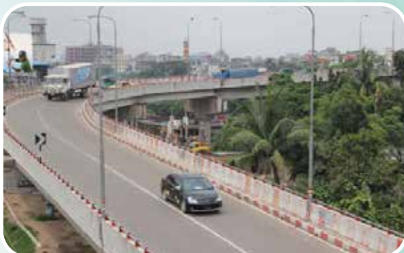
Project Name: Tongi Flyover with Nehemiah Anchored Earth Wall
